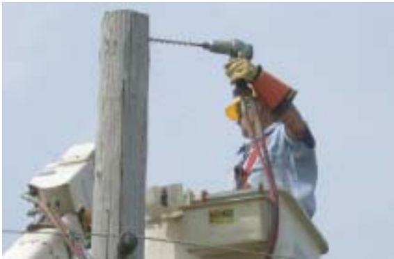
Lineman Kevin Sterland drills a hole in a pole to secure a crossarm.
