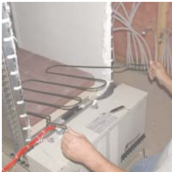
This is the heating element that is used in the ETS furnace. Several of these are placed in between the bricks.
