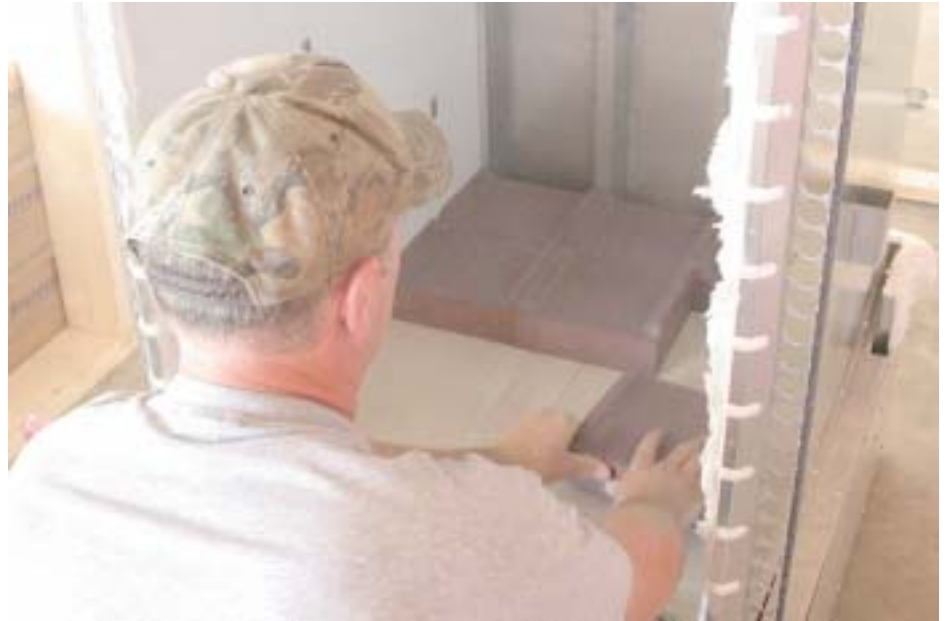
Greg Shaw of Clark Electric Appliance & Satellite, Inc., is installing the ceramic bricks used to store the thermal energy, which can be used later.
